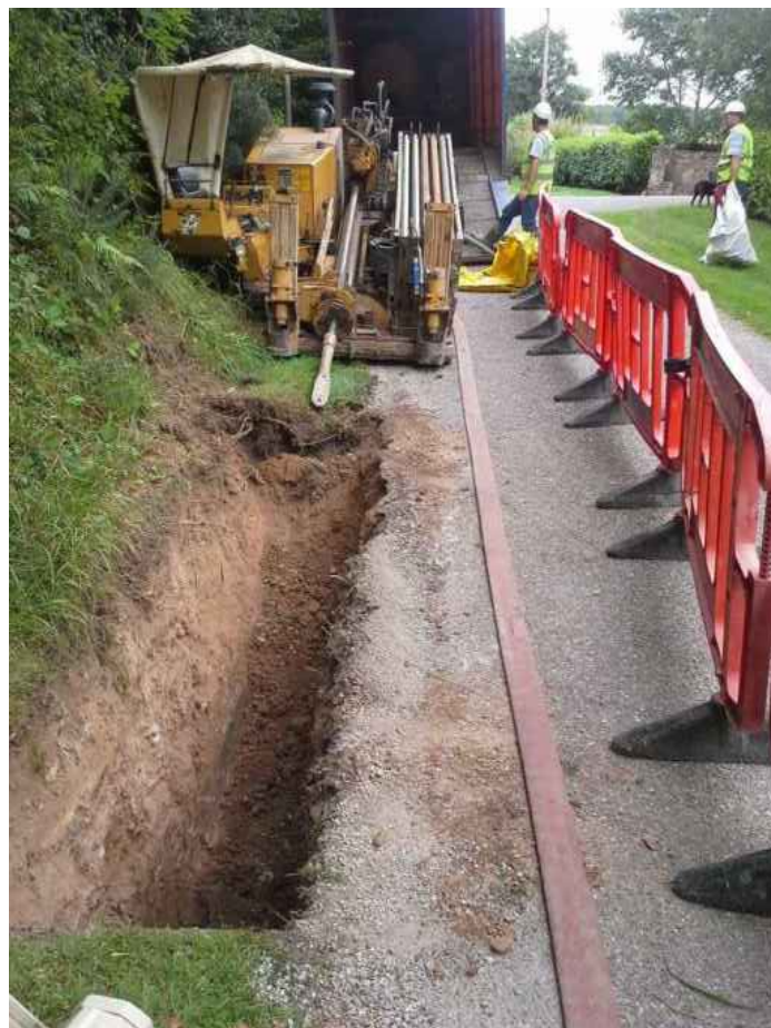
Drilling Rig/Launch Pit
